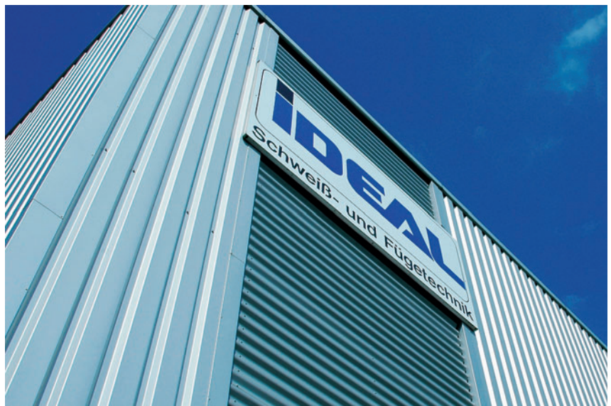
Production plant in Lippstadt
